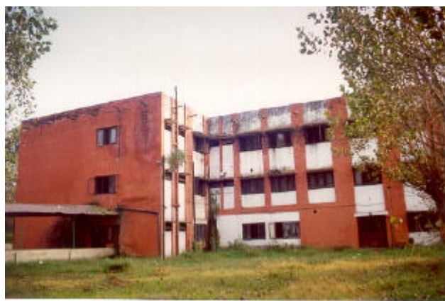
Photo II-1: Brick in cement building
