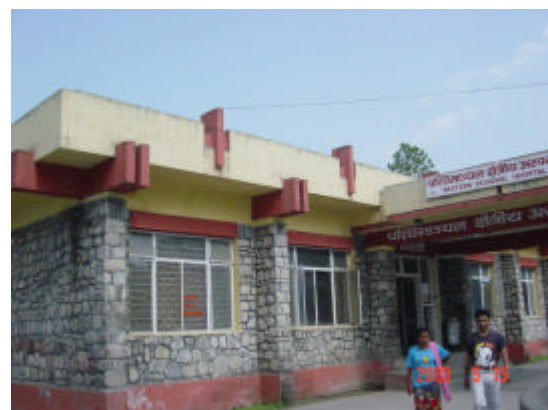
Photo II-2: Stone in cement building
