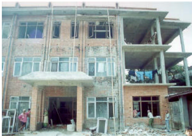
Photo II-3: Ordinary Moment Resisting Frame Building
